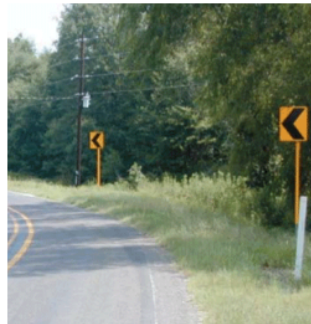
Chevron signs with retroreflective strips on sign posts installed along a curve. Source: FHWA
