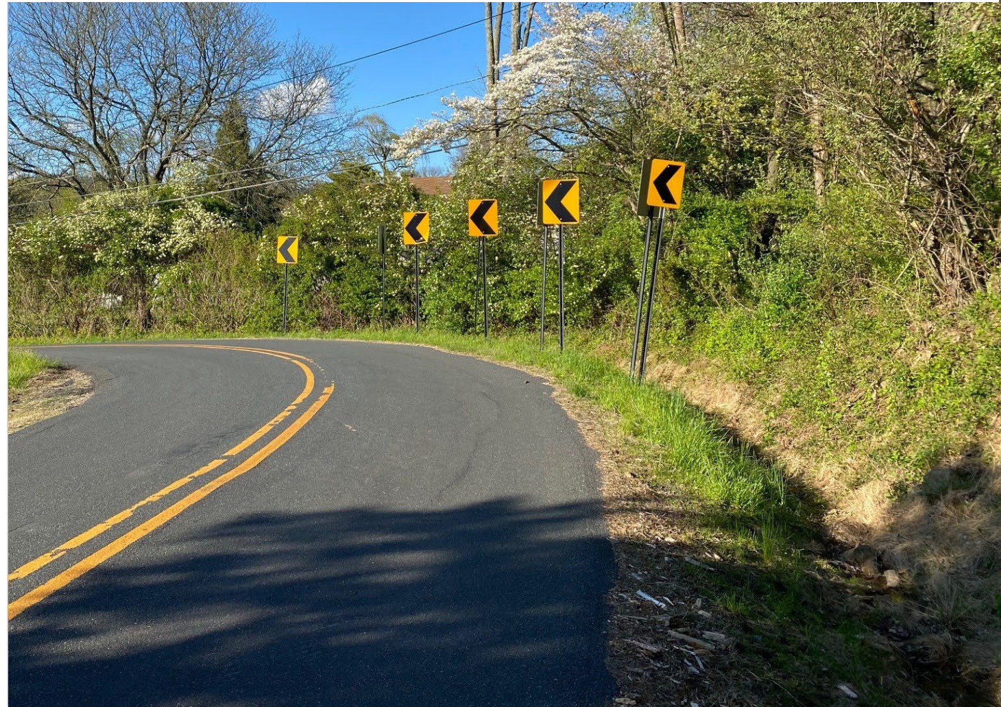
Chevron signs with retroreflective strips on sign posts installed along a curve. Source: FHWA
